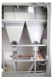
The Kice Pneumatic/Air Make-Up System includes two SV16-8 bag house filters, with modifications and additions.
